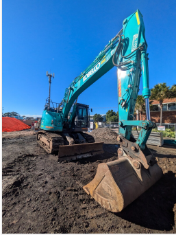
Front Left Corner
